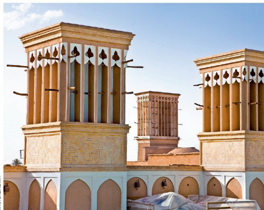
Windcatchers let cooler air flow into houses through a chimney
